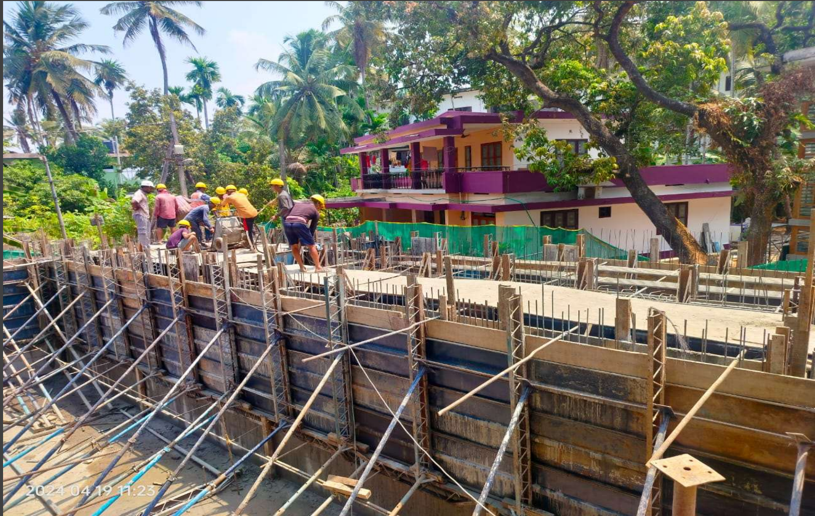
Sump tank side wall RCC
