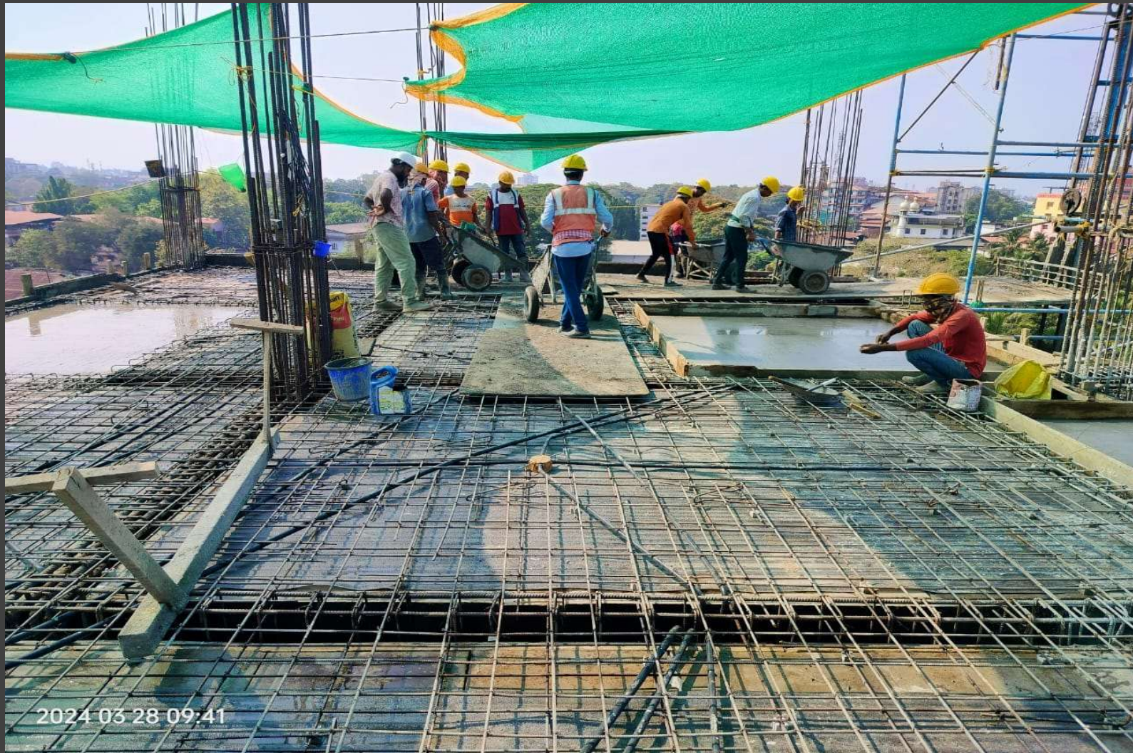
Ninth floor slab RCC
