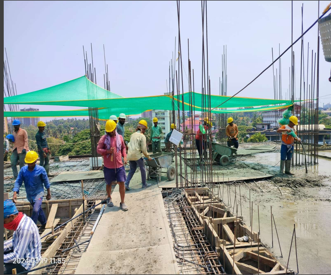
Seventh floor slab RCC
