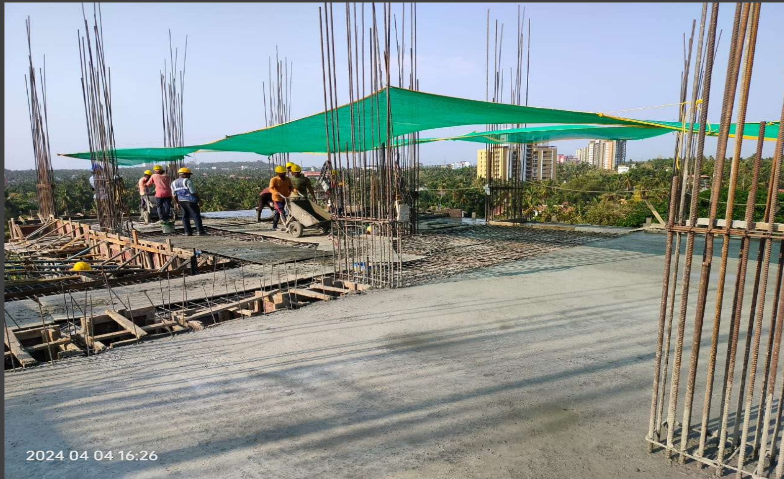
Eighth floor slab RCC
