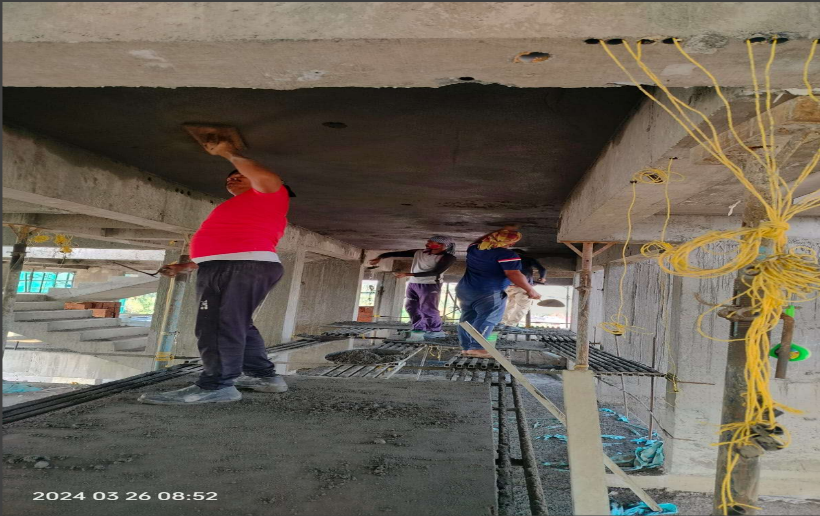
Ceiling plastering – Fourth floor
